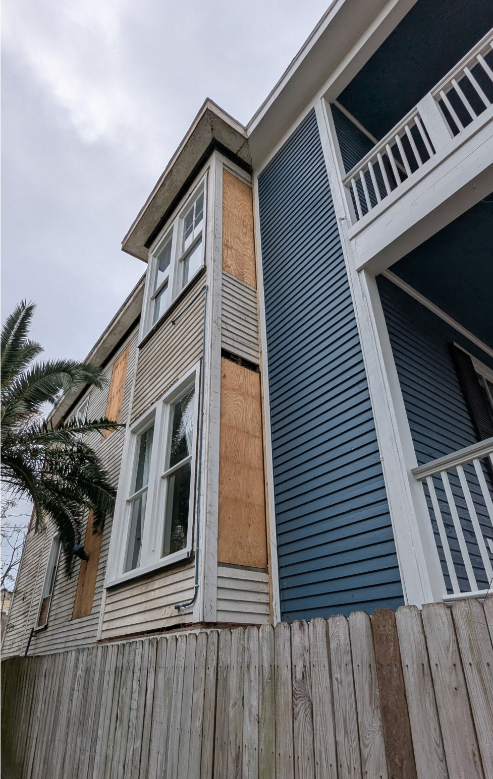
East side: View from the front of the home
