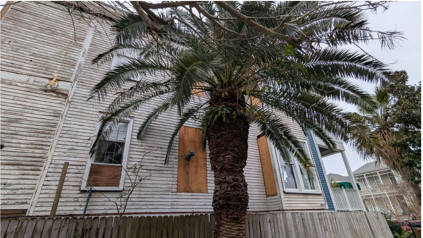
East Side: Back section was previously a covered porch & balcony. Non-historic wood. Enclosed in the 1970s to create apartments.
