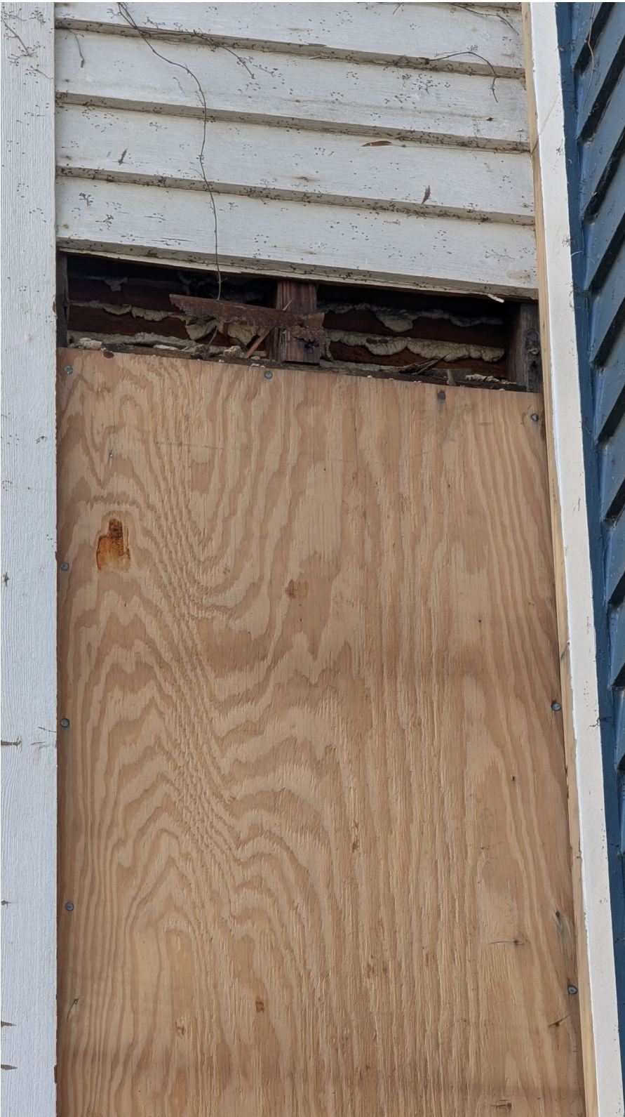
Close-up of plywood and wall
