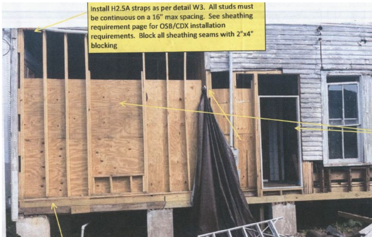
South (Rear) Before Work
