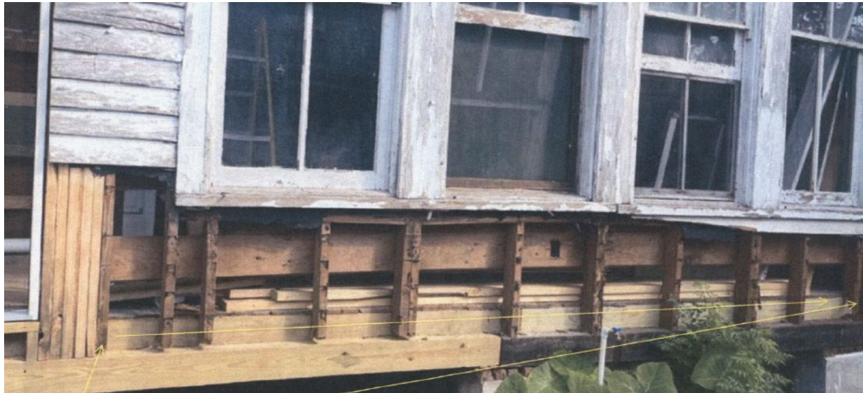
South (Rear) Before Work
