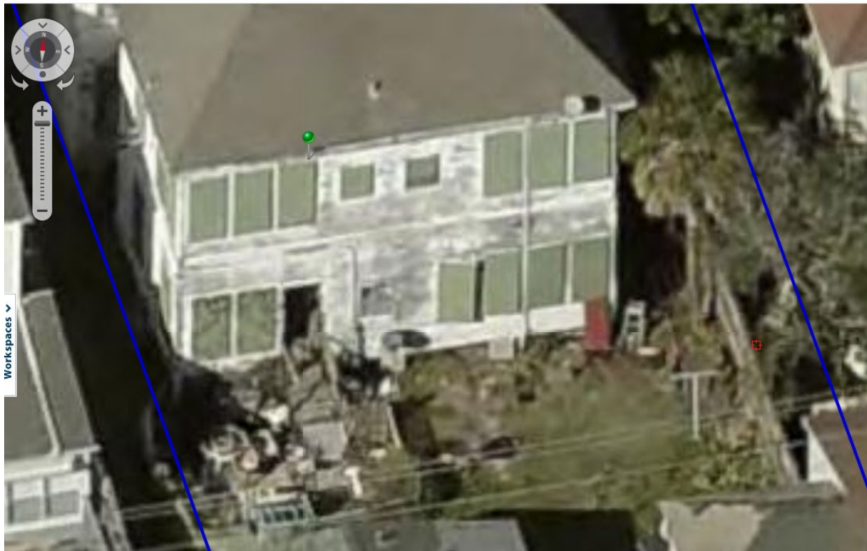
South (Rear) Before Work
