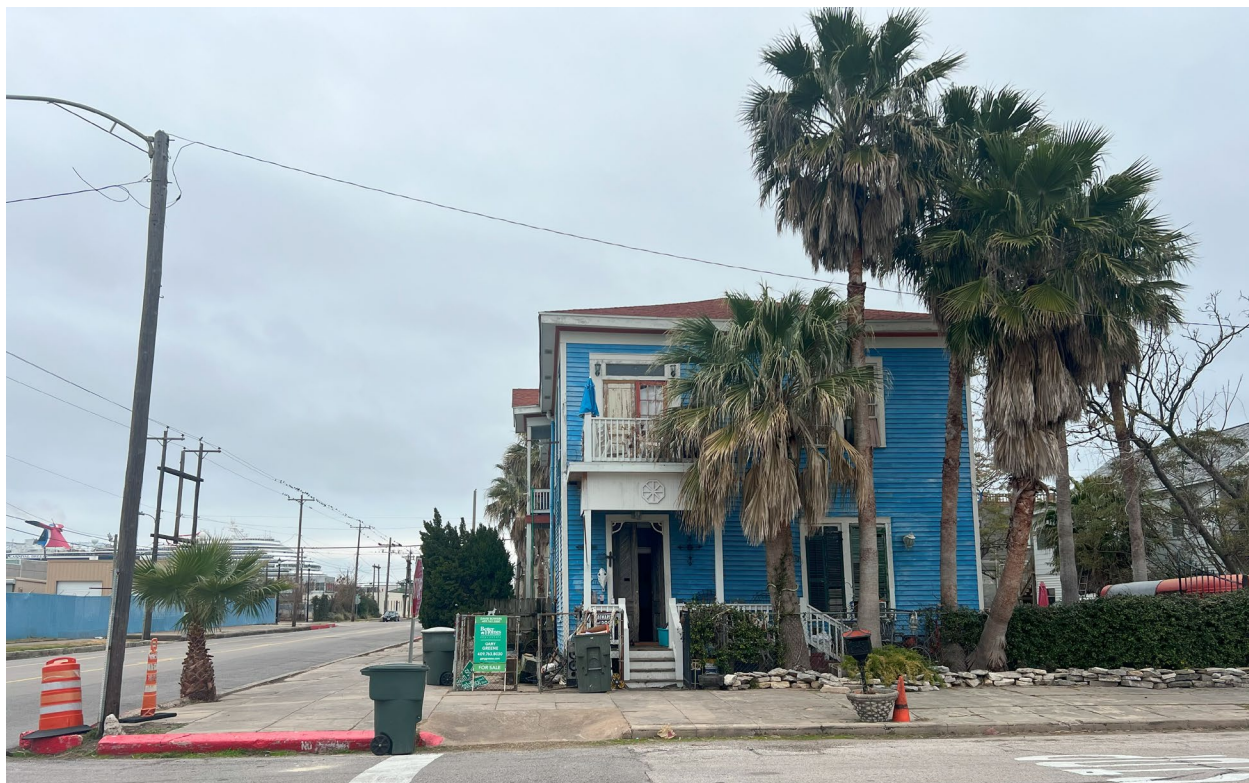
SOUTH ELEVATION – MAIN ENTRANCE
