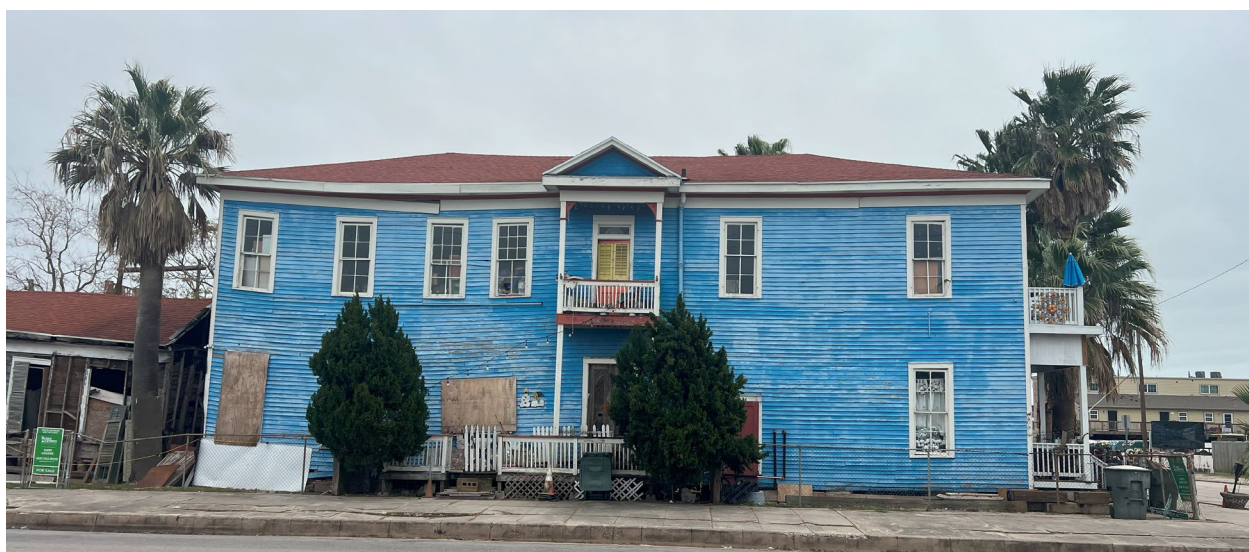
WEST ELEVATION – SIDE ENTRANCE
