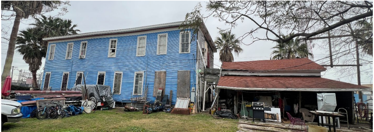
EAST ELEVATION WITH BURNT ONE-STORY STRUCTURE
