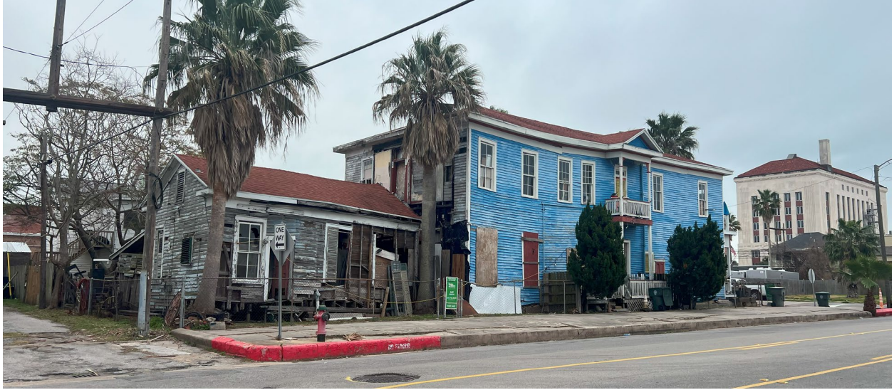
REAR ELEVATION WITH BURNT ONE-STORY STRUCTURE
