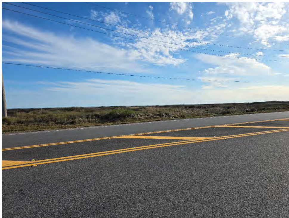
Southerly view of the western portion of the site. January 12, 2026
