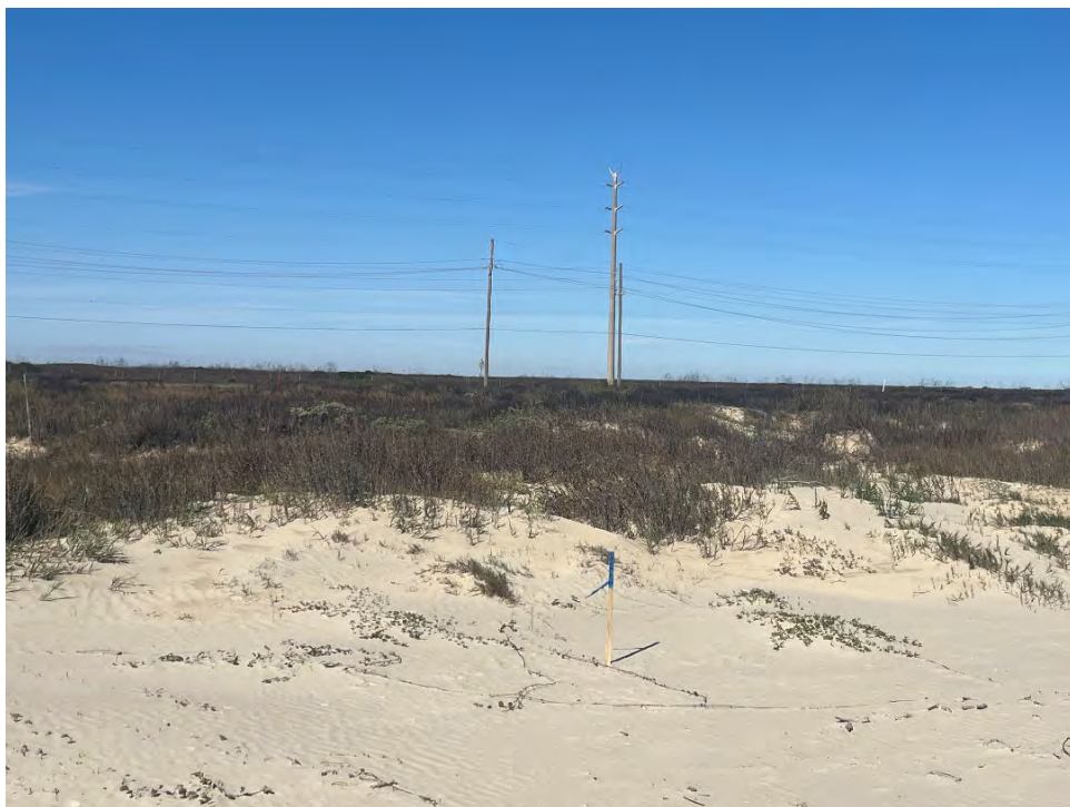
Northerly view near the center of the site. The blue painted stake was one of several that identify the South Toe of Dune 2. The Line of Vegetation was staked but removed by beachgoers. It was recorded with GPS as shown on our layouts. January 12, 2026
