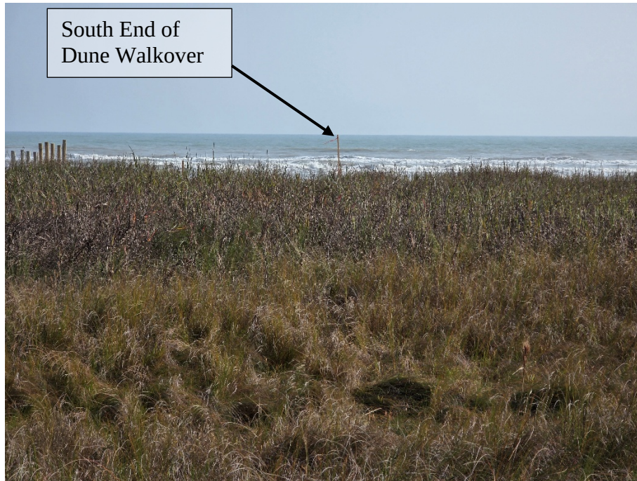
Southerly view along the proposed Dune Walkover alignment as seen from the North Toe of Dune. January 6, 2026
