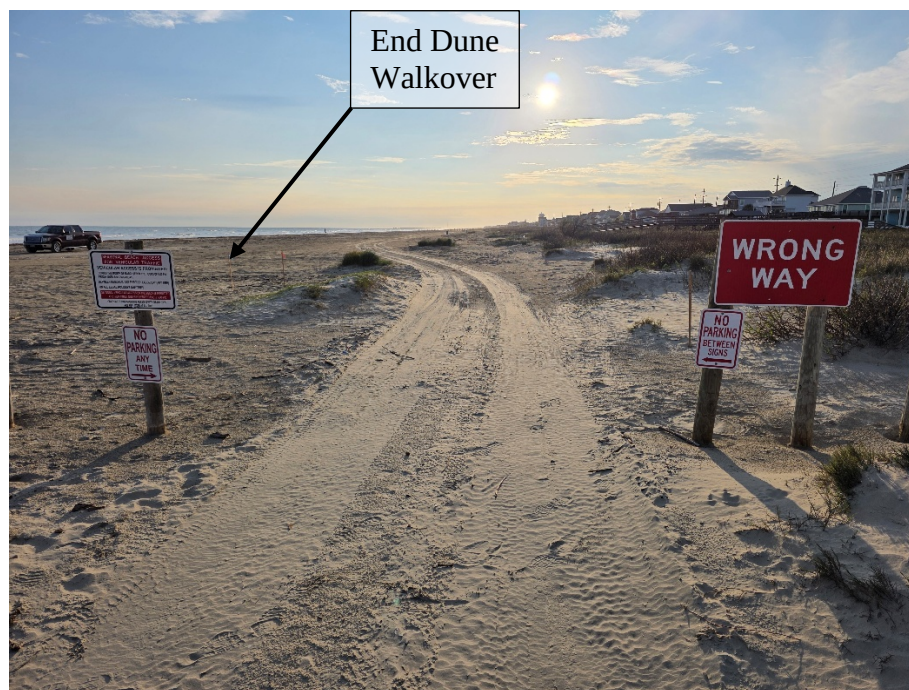
Westerly view at the gap in the bollard line. The gap in the bollard line will be closed and moved closer to the Beach. January 12, 2026
