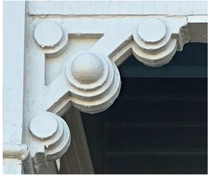
Porch Details, upper & lower: Cloverleaf trefoils in Frieze Brackets (bossing on 2 nd floor) "Bow tie" Chamfered Posts St. Andrew's Cross Guard Rail
