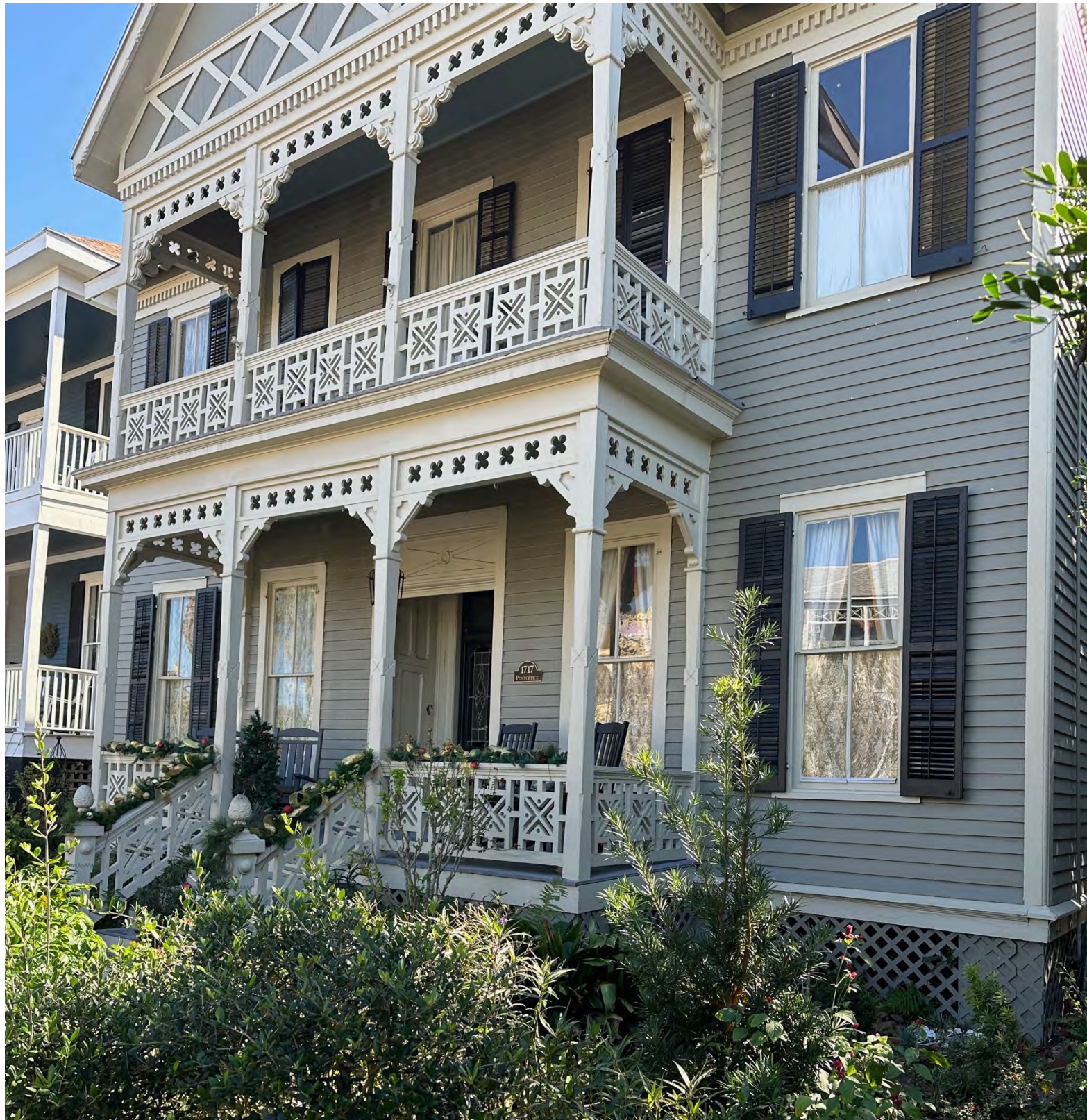
View from Northwest corner of porch at 1717 Postoffice St.
