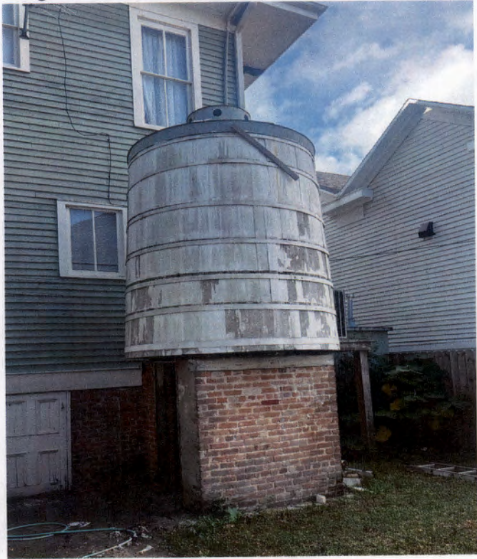
Original Rainwater Cistern, 2116 Avenue N, Galveston, TX”
