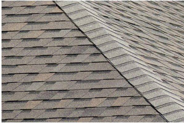
GAF Composite asphalt shingle roof
