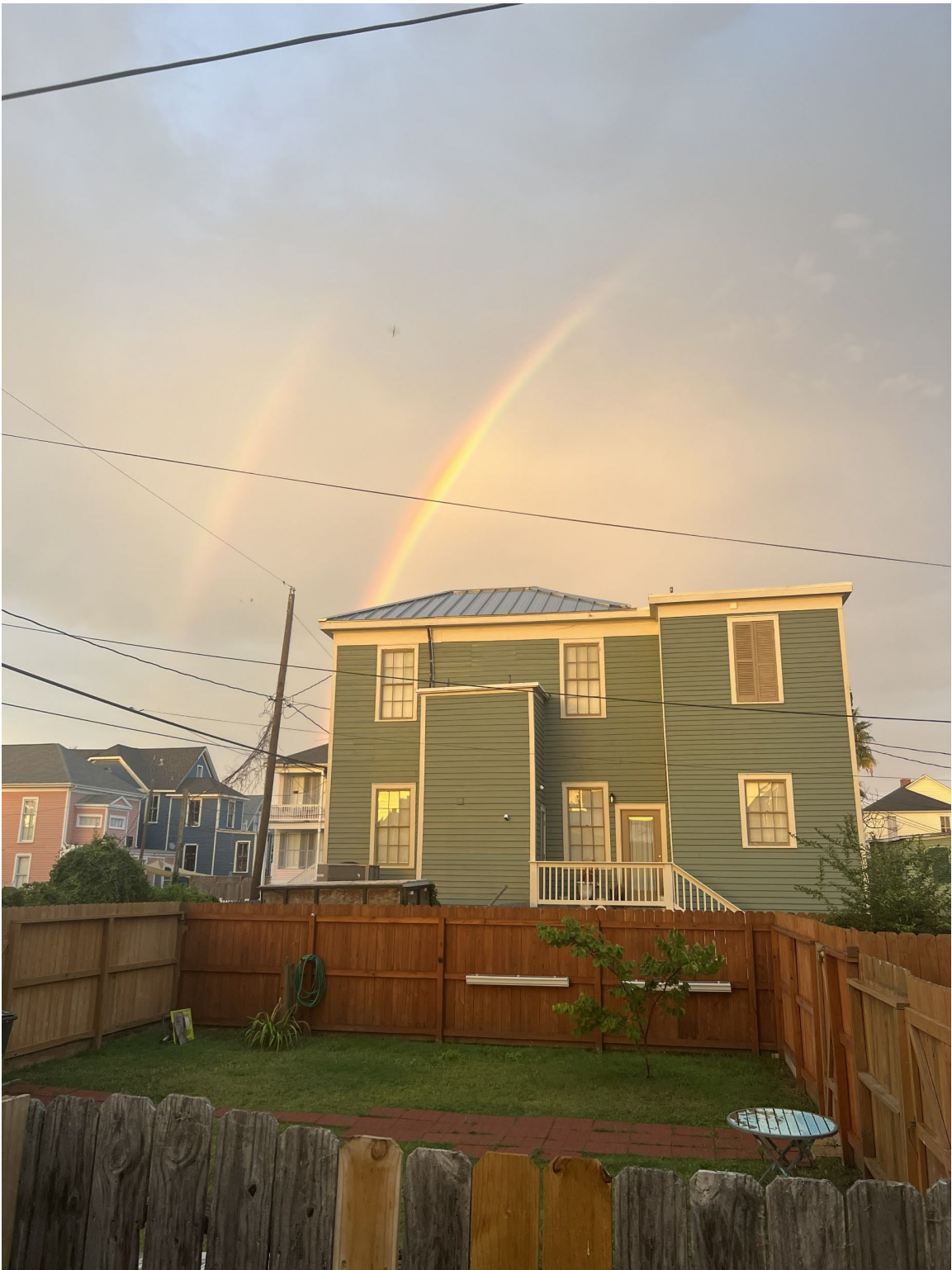
Rear of House
