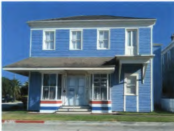
A barbershop now operates at the 1859 William Werner Grocery Building, 1401 Church Street, one of Galveston's oldest surviving corner store buildings.
