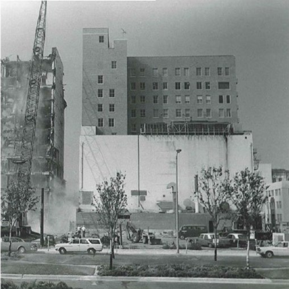
Historic Photo: East Elevation, Looking West
