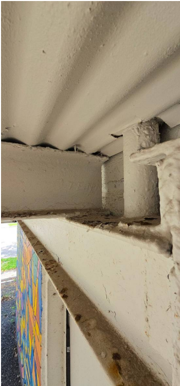
Red- Severe Corrosion present on left side post supporting balcony. Recommend replacement of steel post. Orange- Steel truss has severe corrosion present at time of inspection. Recommend replacement.
