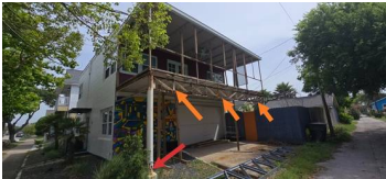
Red- Severe Corrosion present on left side post supporting balcony. Recommend replacement of steel post. Orange- Steel truss has severe corrosion present at time of inspection. Recommend replacement.
