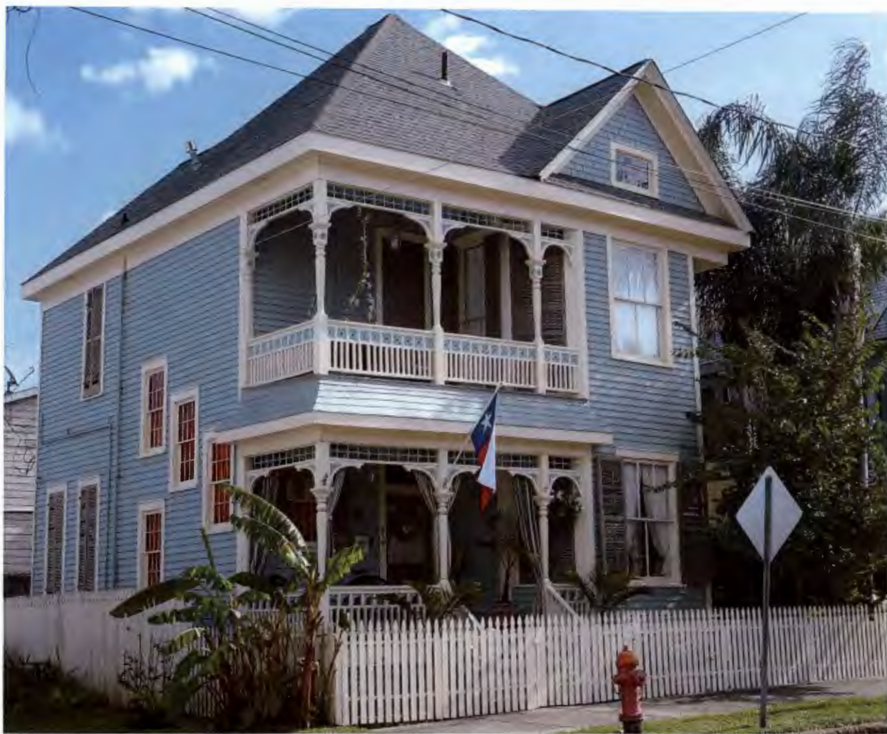
North and west elevations. Unique eight-over-eight windows can be seen on the north elevation. The three windows at staggered heights illuminate the interior double-turned staircase with the fourth window provides light for the original downstairs bathroom. A fifth eight-over-eight window is tucked within the two-bay lower gallery.
