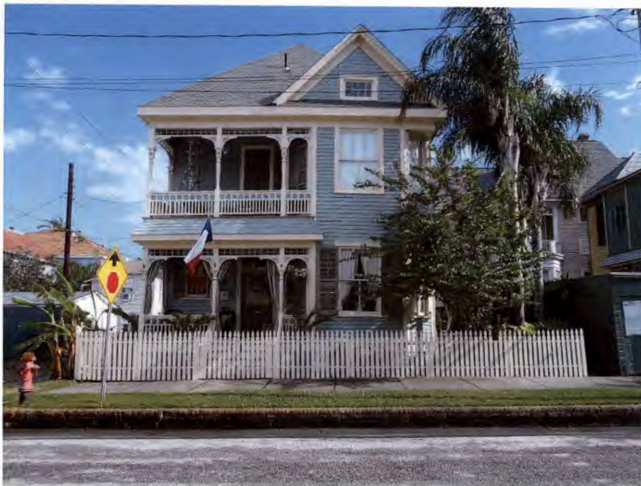
West elevation, the Bonart Tenant House, 514 18 th Street.
