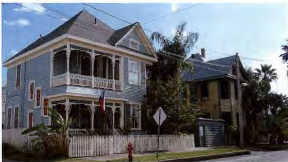
Lot 14, block 437, showing both of the Bonart Tenant Houses, 514 18 th , on the north part of the lot and 1728 Church, on the south part.
