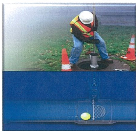
Figure 3: SmartBall Insertion/Extraction
