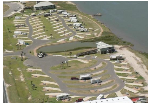
Aerial of MBNP campground
