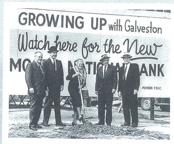
Moody National Bank groundbreaking
