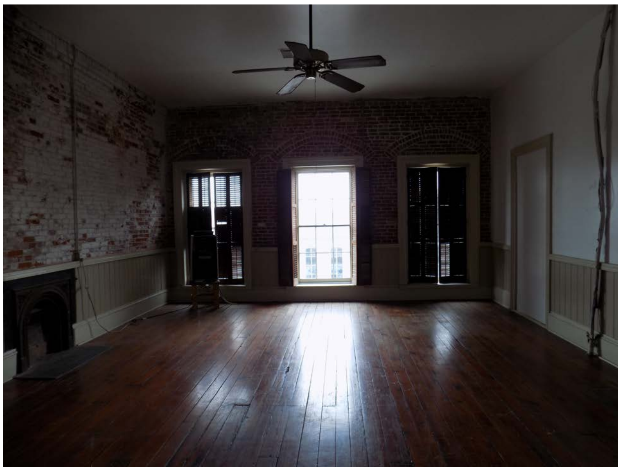
Photo 20: View of Front windows with shutters. Note: The original shutters will be repaired as required and a layer of Tung oil hand applied. The window sash weight cords will be replaced. Weather-stripping will be added.
