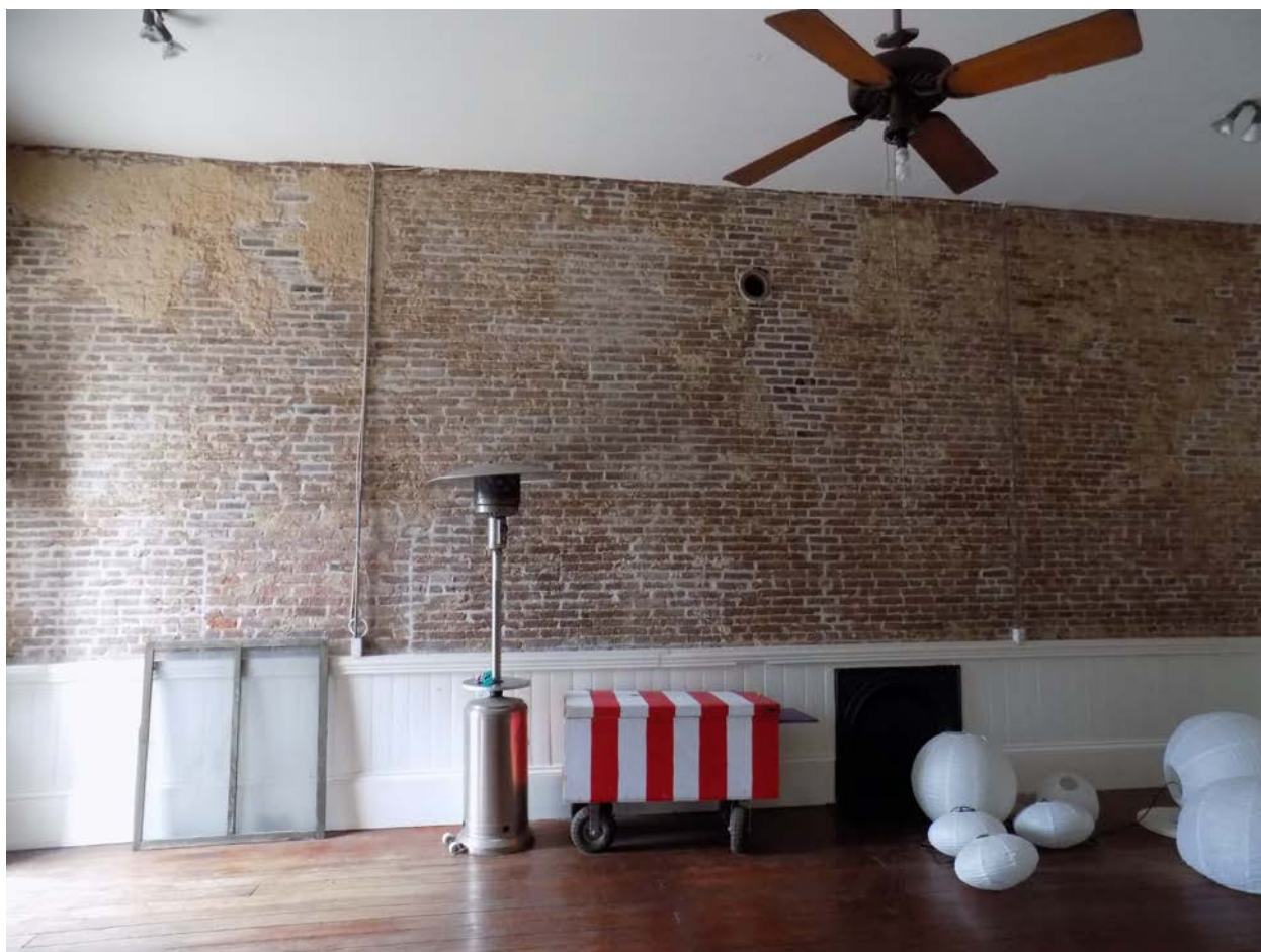
Photo 12: View of West exposed brick wall in apartment 202.
