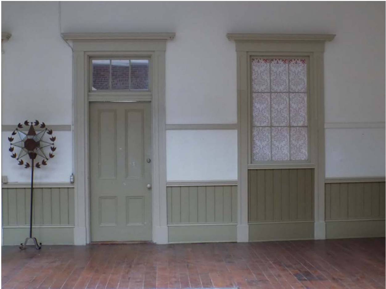
Photo 5: View of Existing typical door and window casing. Note: Existing trim will be retained, cleaned, and painted.
