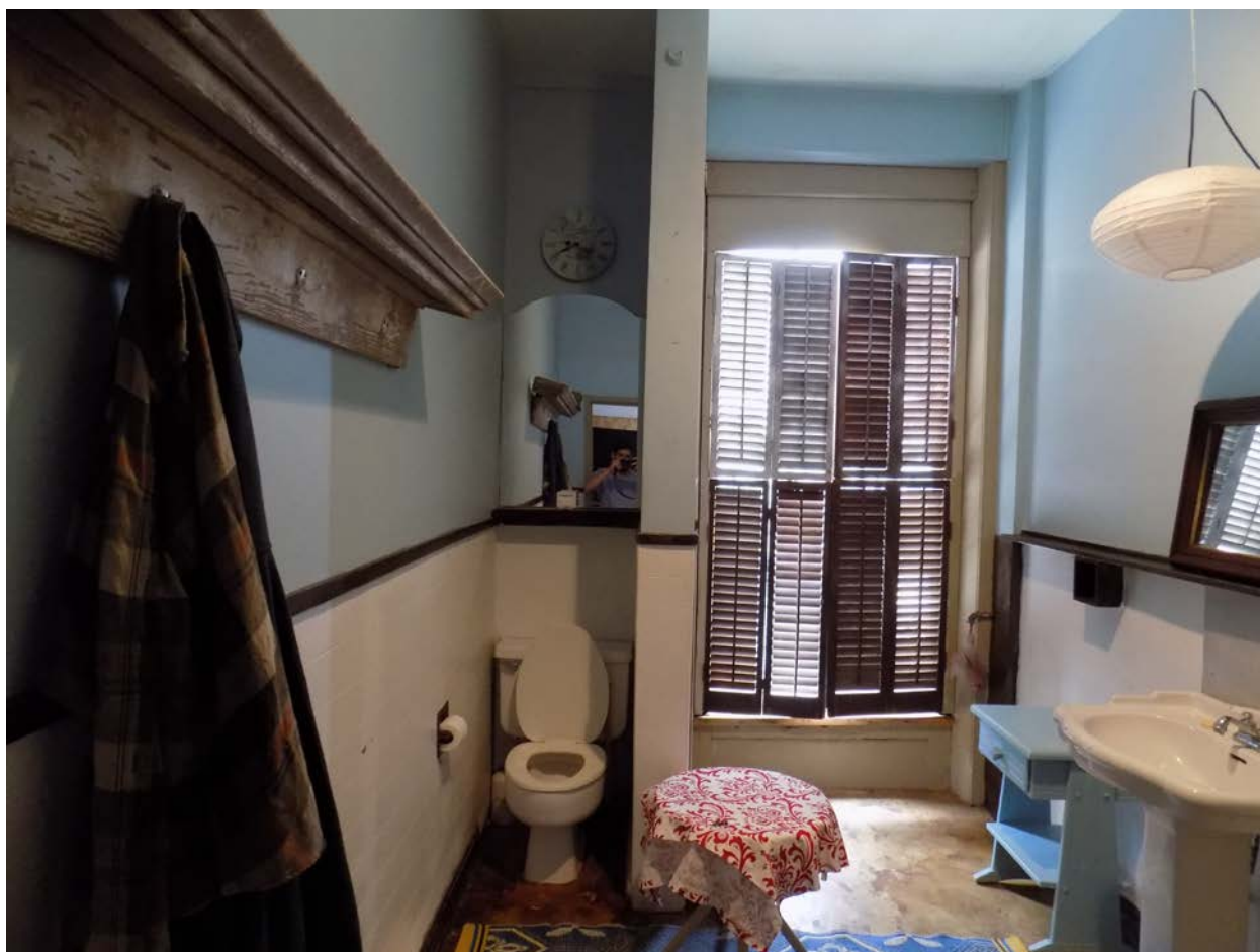
Photo 13: View of Existing bathroom in apartment 203.
