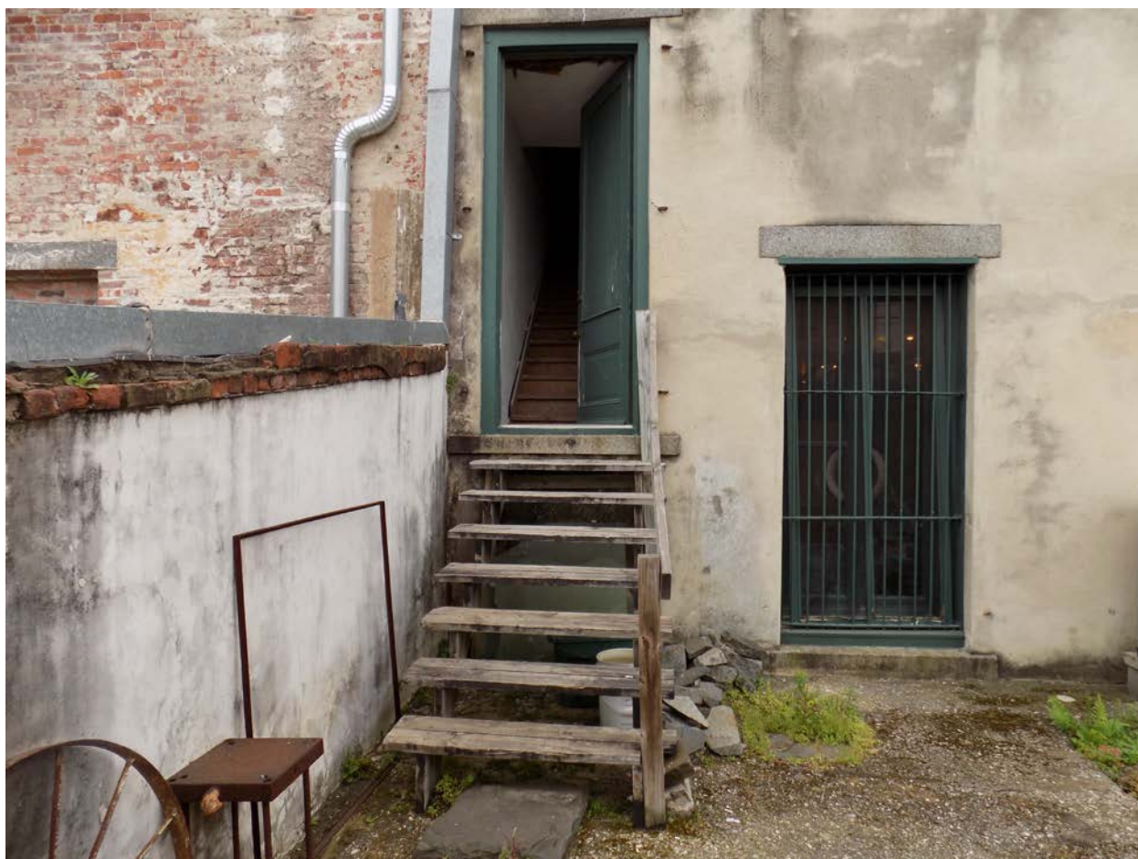
Photo 22: View of Exterior north elevation of existing stair. Note: New hot dipped galvanized stair will be constructed to replace the wooden stair.
