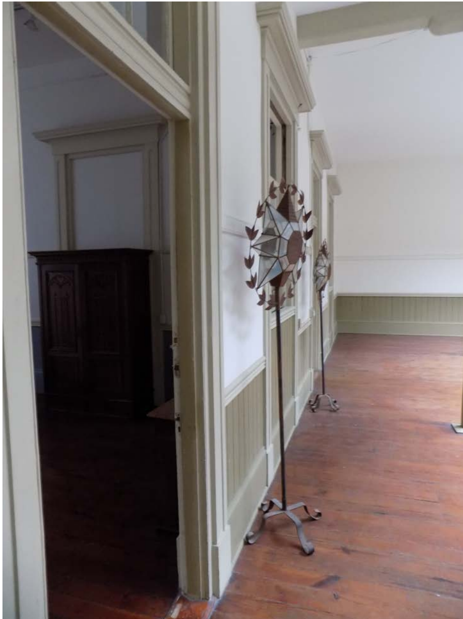
Photo 7: View of Existing demising wall between atrium and front apartment unit 201.
