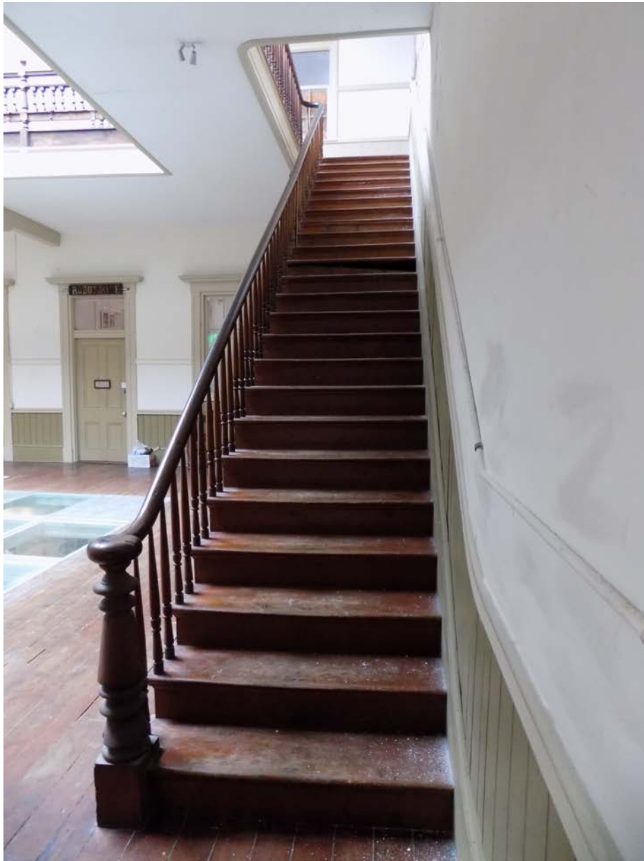
Photo 2: View of existing second floor staircase and balustrade.
