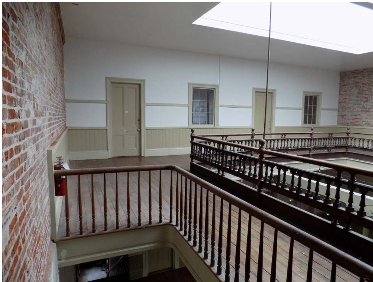
Photo 17: View of Existing demising wall between atrium and front apartment unit 301. Note: The bathroom kitchen will be added in the corner. A raised floor will be installed to allow plumbing drain lines to be installed above the existing floor and not drop down into second floor ceiling area. The window and trim will remain exposed in the bathroom. (Same condition will occur in apartment 302)
