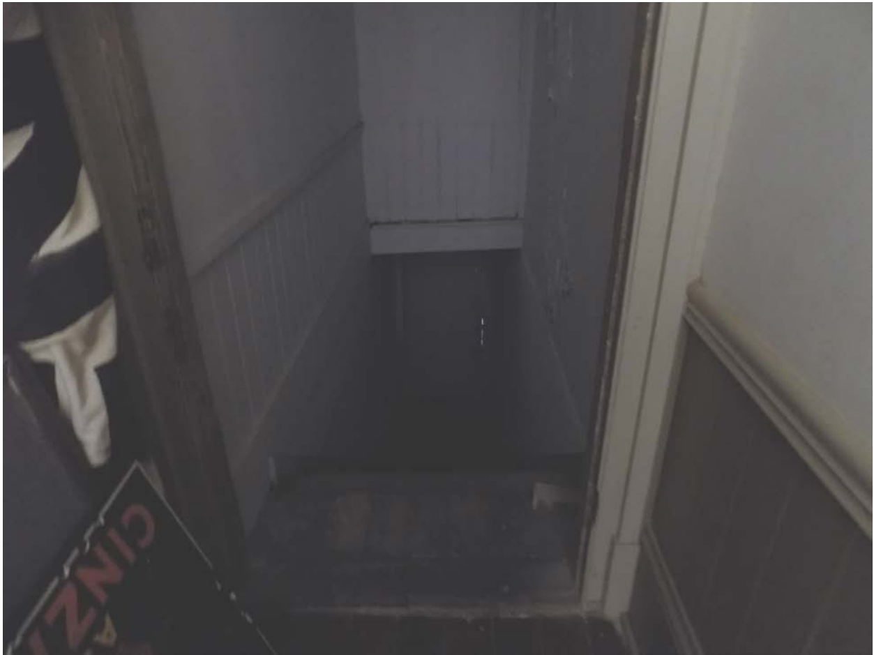
Photo 16: View of Existing north stair to exterior at first floor, currently no light is in this stair well. This will become a part of the fire stairs.
