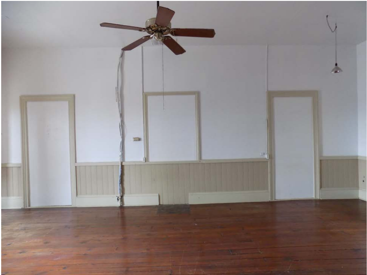
Photo 19: View of Existing demising wall between apartment 301 and 302.
