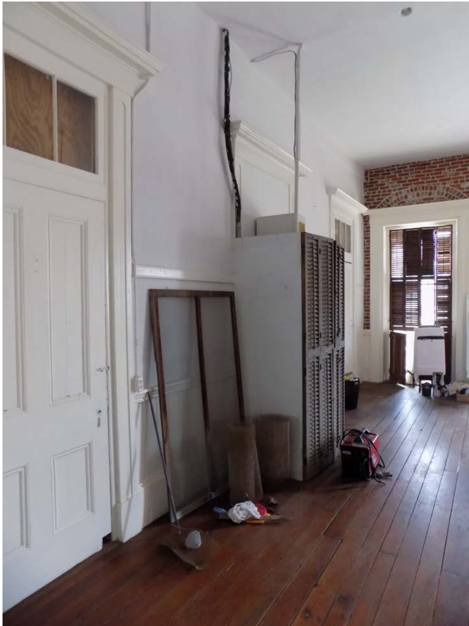
Photo 9: View of Existing demising wall between apartment 201 and 202.
