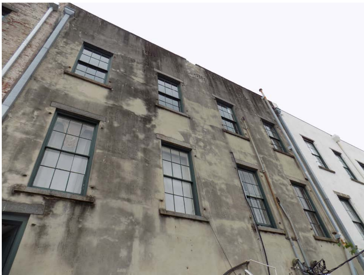
Photo 23: View of Exterior north elevation wall. Note: A hot dipped galvanized frame support for the HVAC compressor units will be installed above the first floor openings. Compressors must be installed at least 7 feet above surrounding grade to comply with FEMA flood elevation requirements. Roof is pitched and does not offer an optional location for placement.
