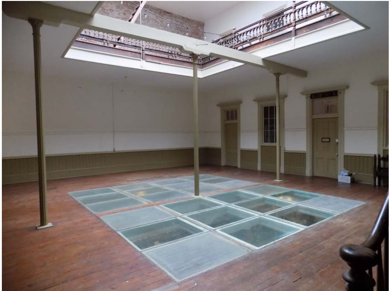
Photo 3: View of Second floor atrium with glass floor. Note: A new 1 hour fire rated wall will be added to enclose the first floor and second floor. The wall will be held back from the existing second floor stair balustrade. Double doors from the landing into the atrium will be on magnetic hold open devices to allow doors to remain open except when building goes into alarm. Door trim will be simplified version of existing door casing.
