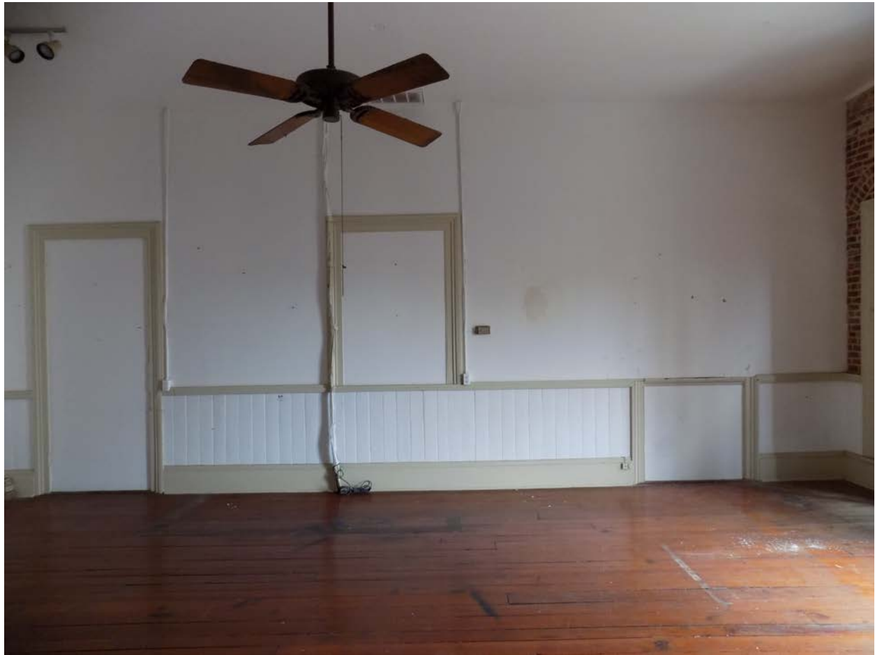
Photo 18: View of Existing demising wall between apartment 301 and 302. Note: The bathroom and kitchen will be added in the corner. The original door was previously removed and in filled with drywall. The trim remains. The wall will be furred out to encapsulate a portion of the historic trim. The trim will remain for future renovations. It is necessary to partially encapsulate this one opening to accommodate new bathrooms and kitchens.
