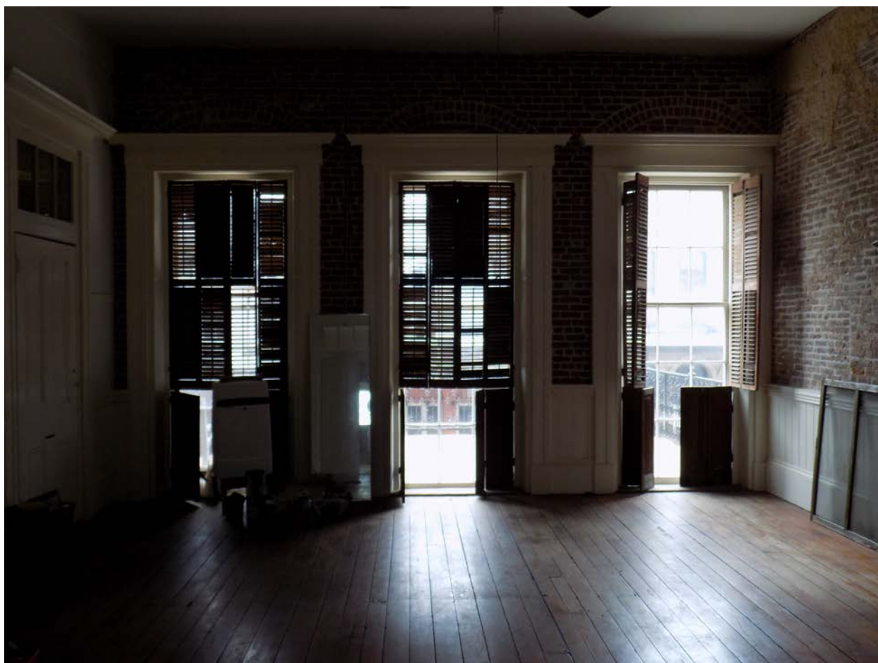
Photo 10: View of Front windows with shutters onto balcony.
