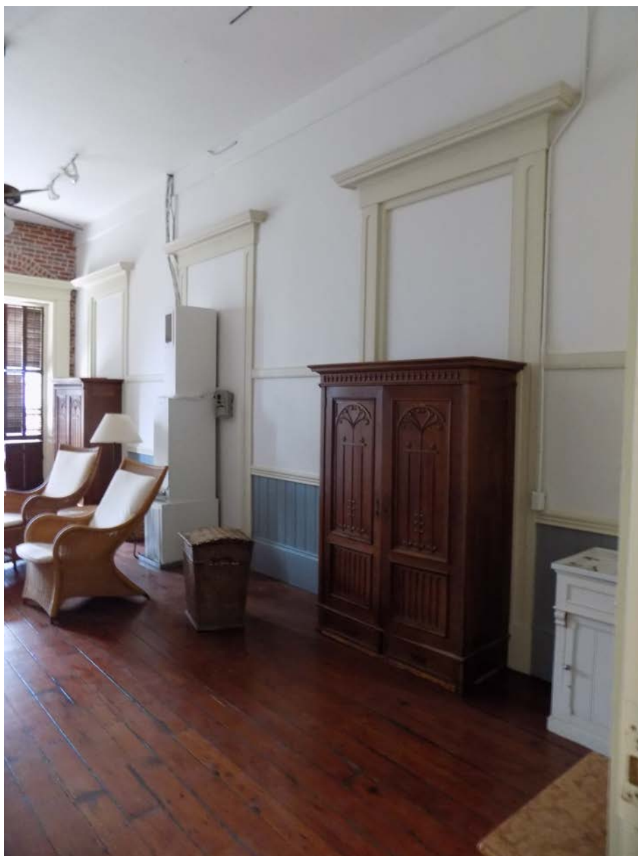
Photo 8: View of existing demising wall between apartment 201 and 202.
