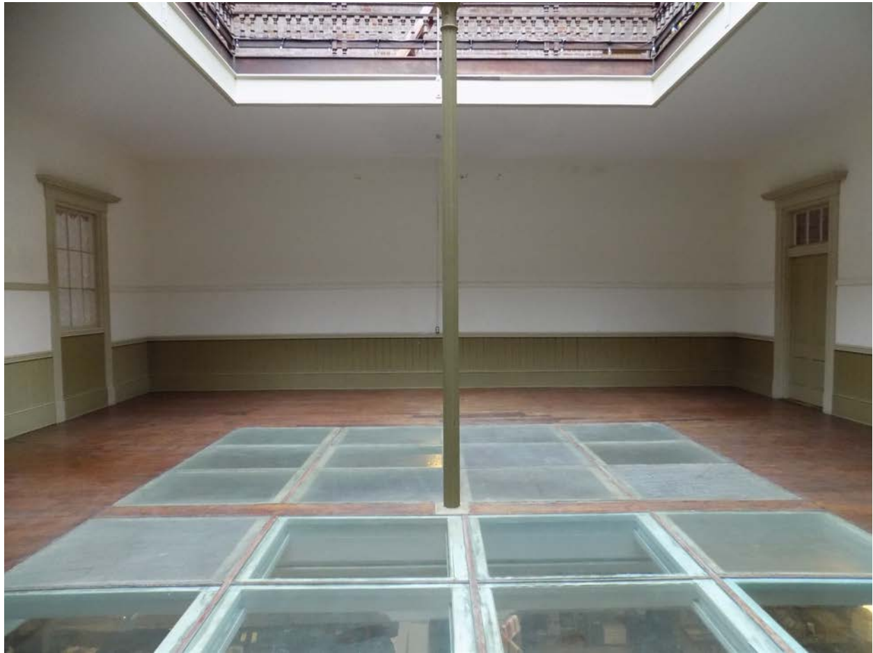
Photo 6: View of Second floor atrium looking west. Note: A new wall will be added to align approximately 3” back from edge of glass floor and balcony above. The new wall base trim will align with base of existing trim without shaped profile detail. No wainscot will be installed on new wall. New door and window trim will be simplified version of existing trim corresponding to width. Doors will not have transoms. The decorative hood detail will be omitted over new doors and window.
