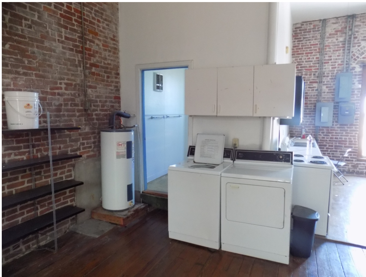
Photo 29: View of existing kitchen and restroom in apartment 303.
