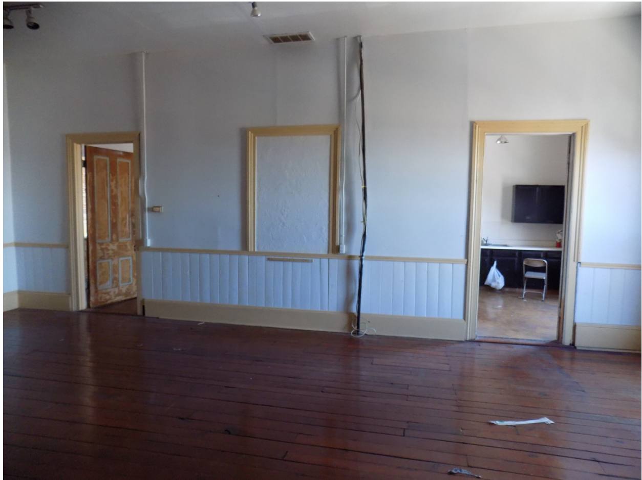
Photo 30: View of existing wall in apartment 303.
