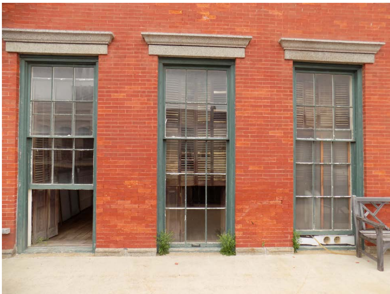
Photo 11: View of Exterior balcony windows.
