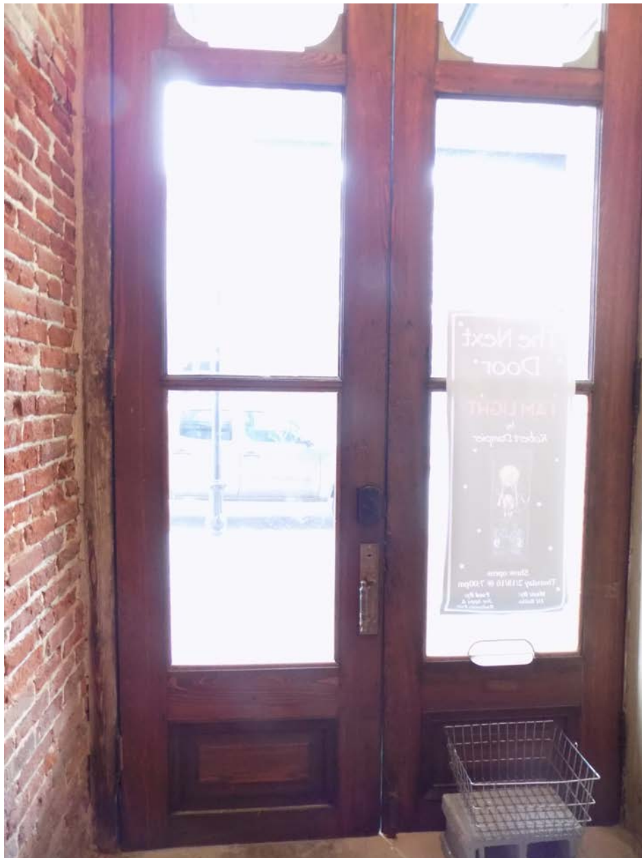
Photo 25: View of Existing interior of Strand doors. Note: Doors will be repaired and hand rubbed with Tung oil.
