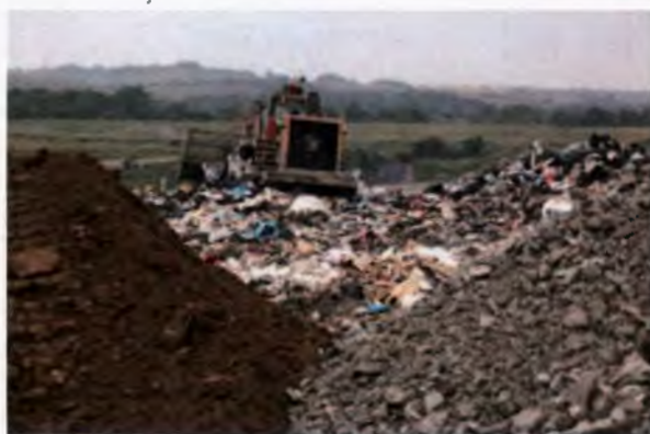
Figure 9. Landfill - Our landfill operations are staffed by highly trained environmental and landfill engineers
