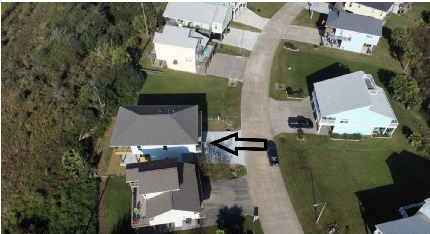
Aerial looking North
