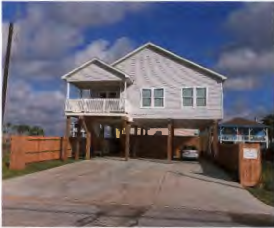
Front View - porch is 32' from street
