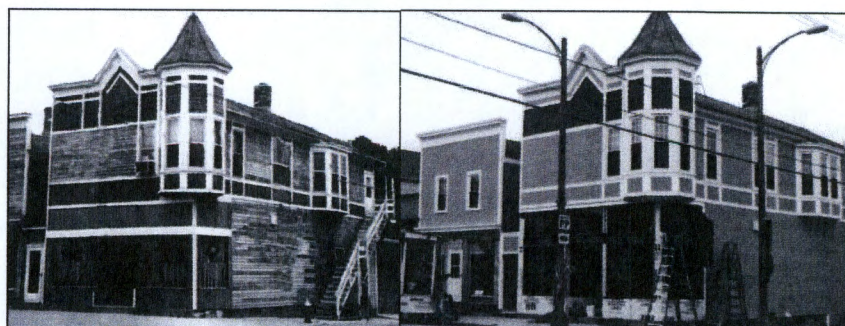
Due to extreme deterioration, the original wood siding on this building was replaced with fiber-cement siding. Note that the original trim pattern and siding width were replicated properly.
