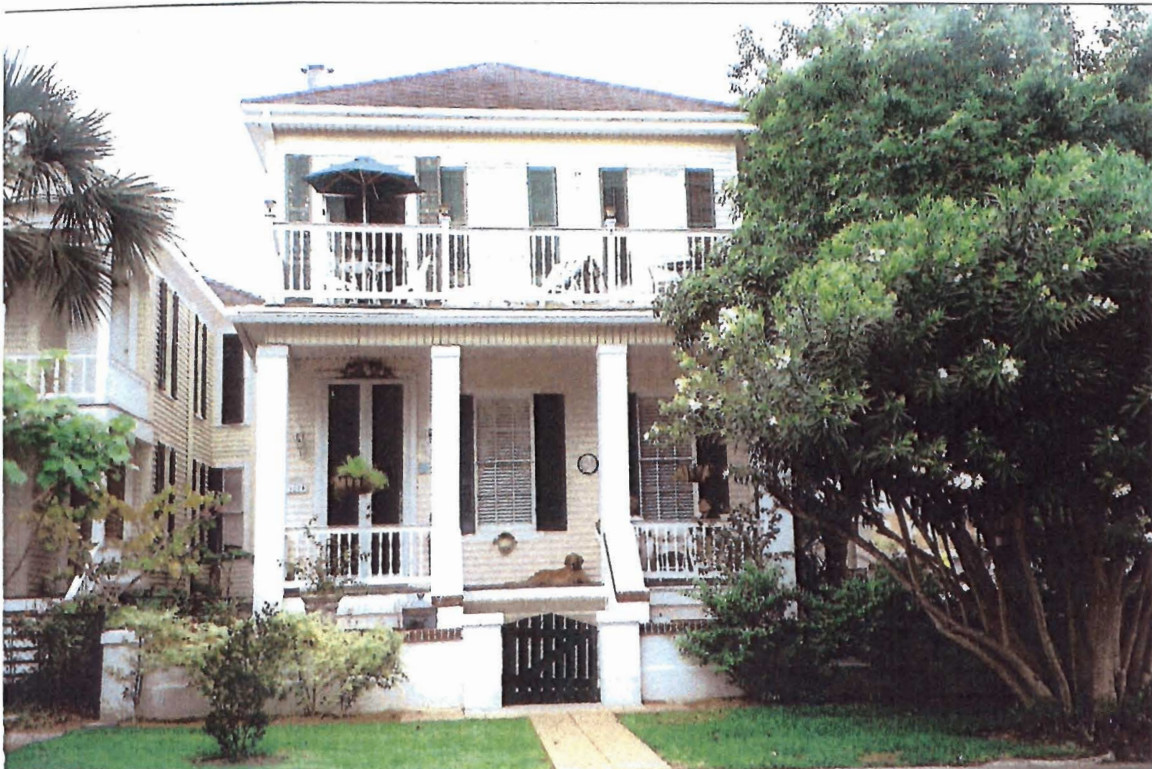
Before Hurricane Ike
